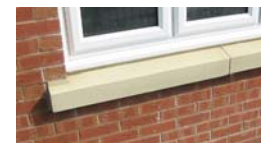
Cast stone cills and lintels
